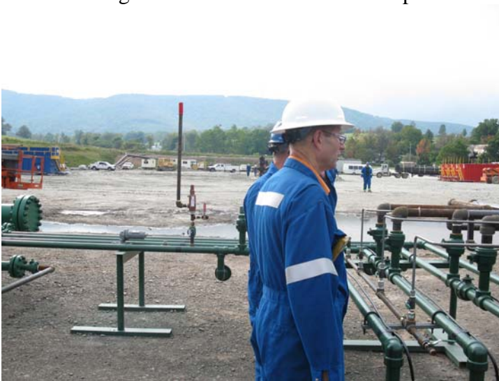
Gas "treatment" is minimal as gas is very clean, only needs dewatering and then sent to pipeline.
