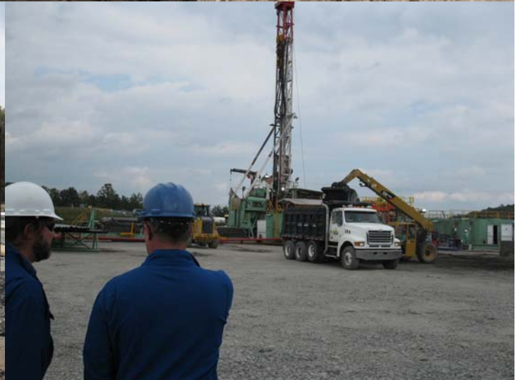
Drilling rig and drill cuttings being loaded
